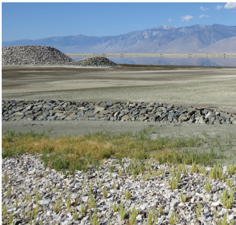
FIGURE 4-12 Use of cobbles and boulders at Owens Lake as part of the Land Art Project, with cobbles used along trails to provide enhanced public access. The cobbles trap seeds and sand, providing sites for the establishment of native vegetation.
