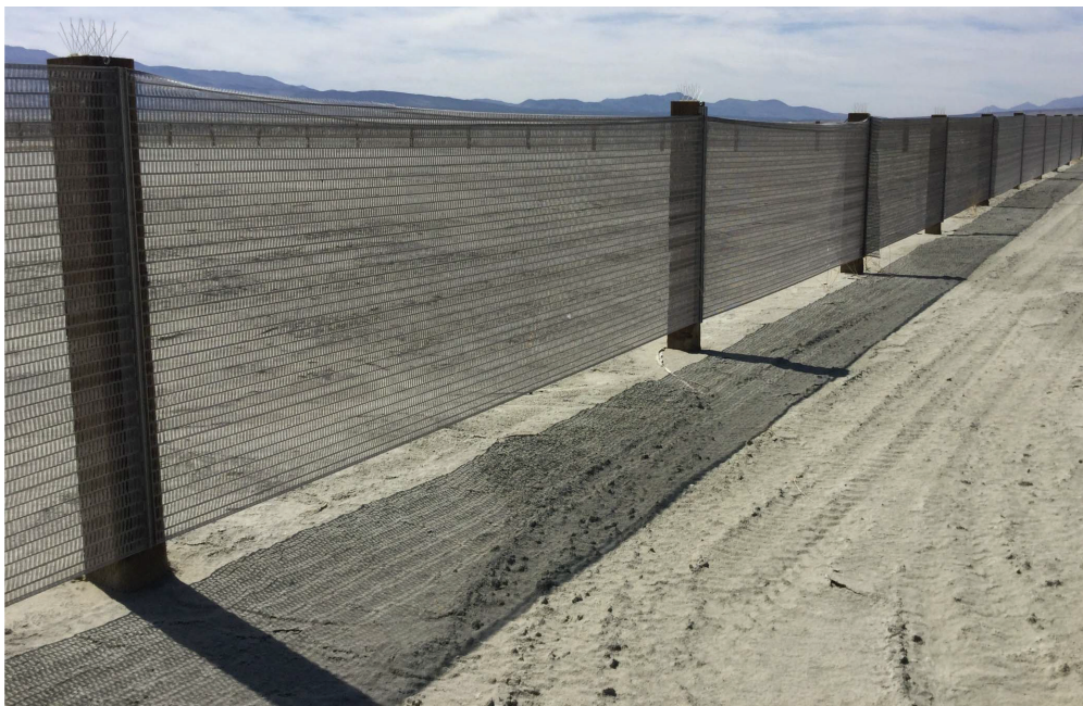
FIGURE 4-13 Sand fence at Owens Lake. SOURCE: Schaaf, 2019.
