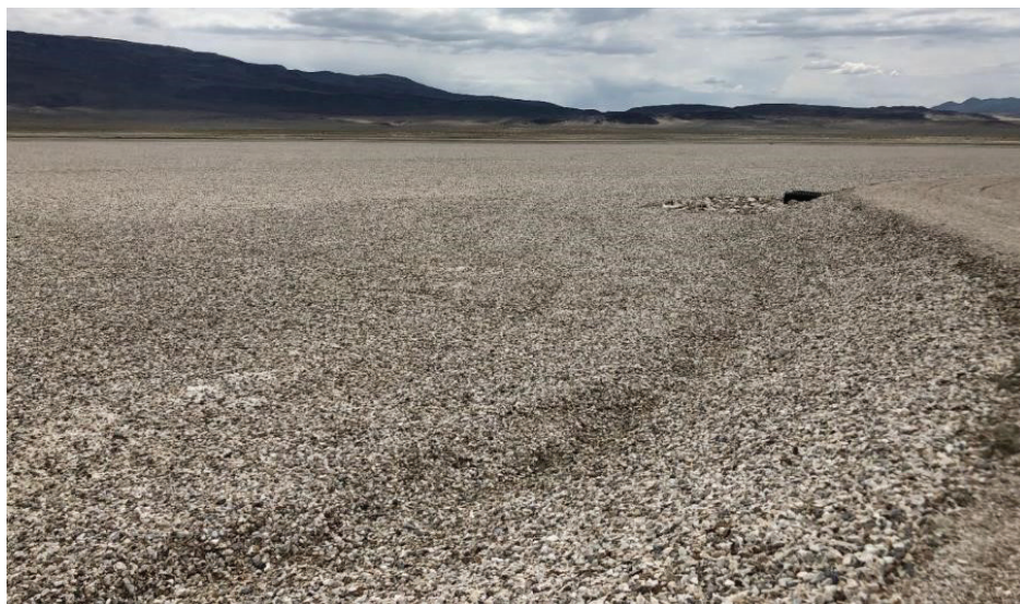
FIGURE 4-9 Dust control using the gravel BACM. SOURCE: Photo courtesy of Stephanie Johnson, National Academies.
