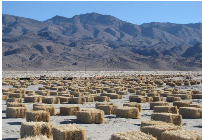
Figure 6-6: Straw Bale Array in the Keeler Dunes Dust Control Project (January 2015)
